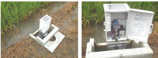
**Fig.2 Remote controlled valve at a water inlet of a paddy field plot.**
