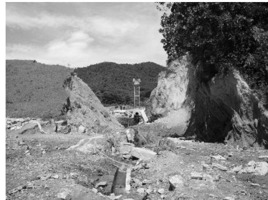
Picture 1: KE 2/20 REC dam failure
